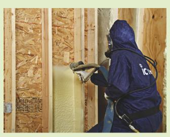
Pictured is Icynene's new LD-50 spray-foam insulation. McCutcheon and his team use spray-foam in many applications, especially to seal up roof rafter planes.
